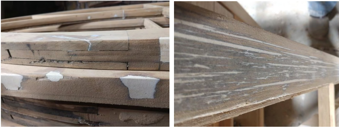
Photos of same window showing in-progress repair with epoxies and wood fillers.
