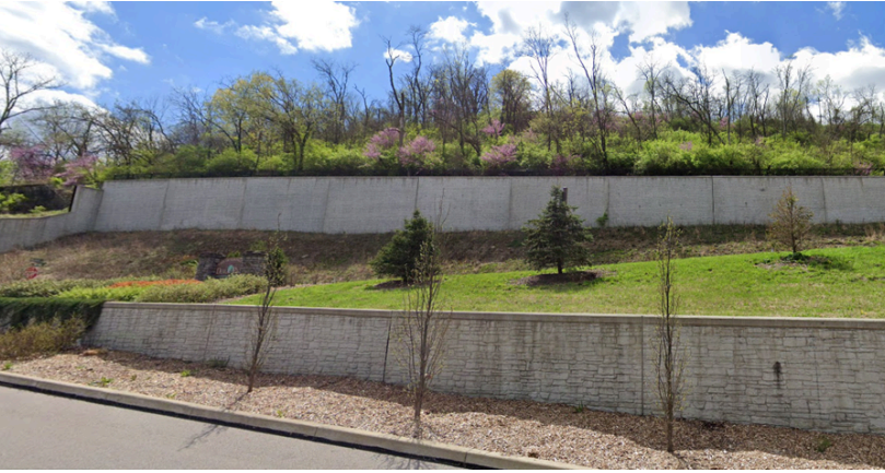
Devou Park Drive Stabilization
